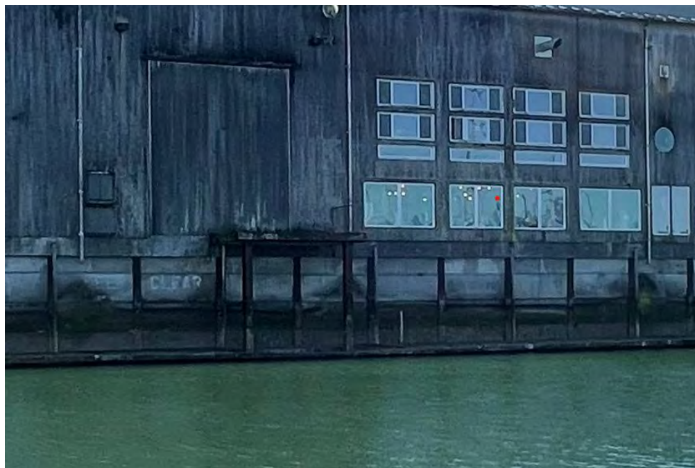
Photo 3. Typical view of retaining wall showing piles and support wall.
