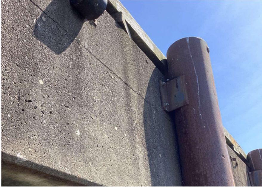
Concrete Cap Exterior Face
