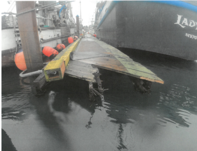
Photo 12: West end of Dock E/F
