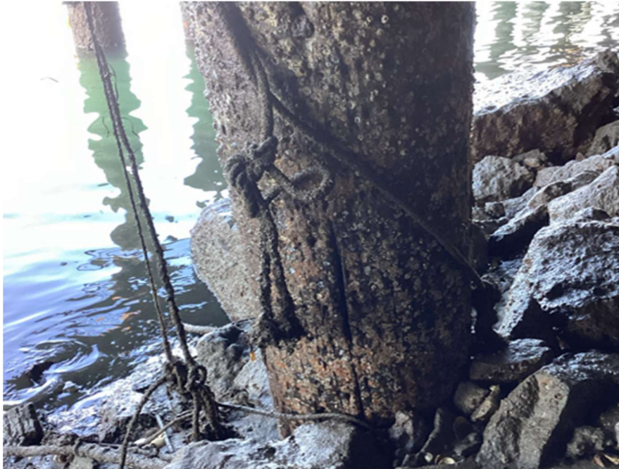
Timber Pile Checking
