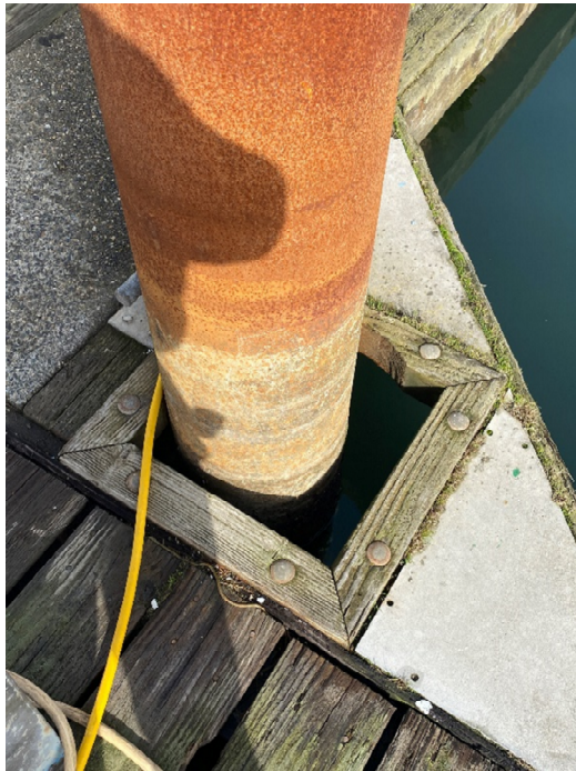
Photo 6: Rub block at piles
