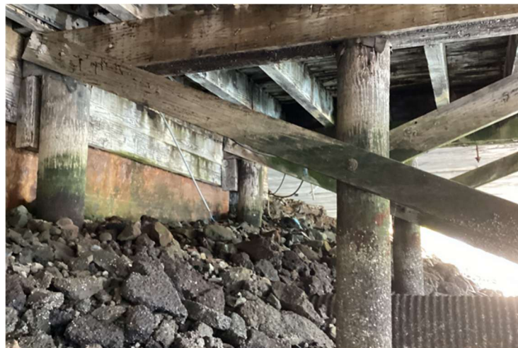
Timber Pile and Cap
