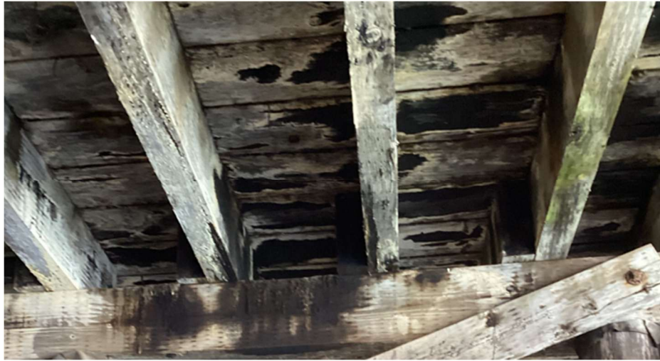
Underside of the Timber Deck
