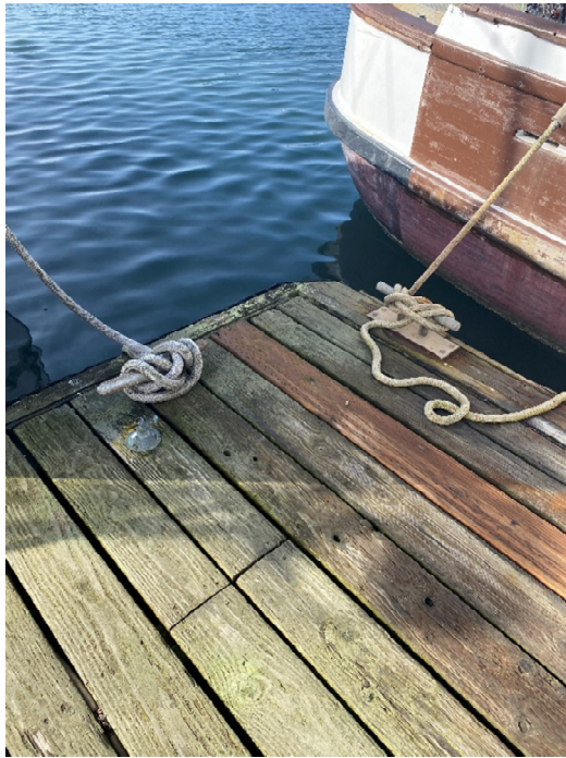
Photo 8: Typical condition of mooring hardware
