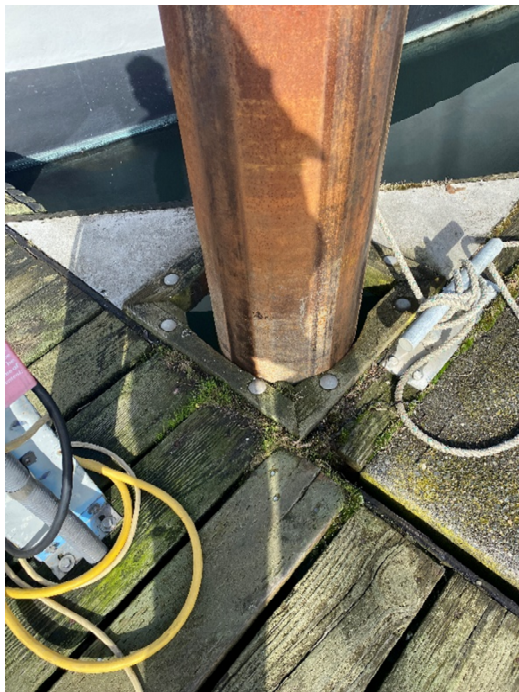
Photo 7: Rub block at piles
