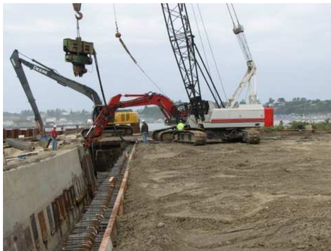
Driving Sheet Piling at the Terminal
