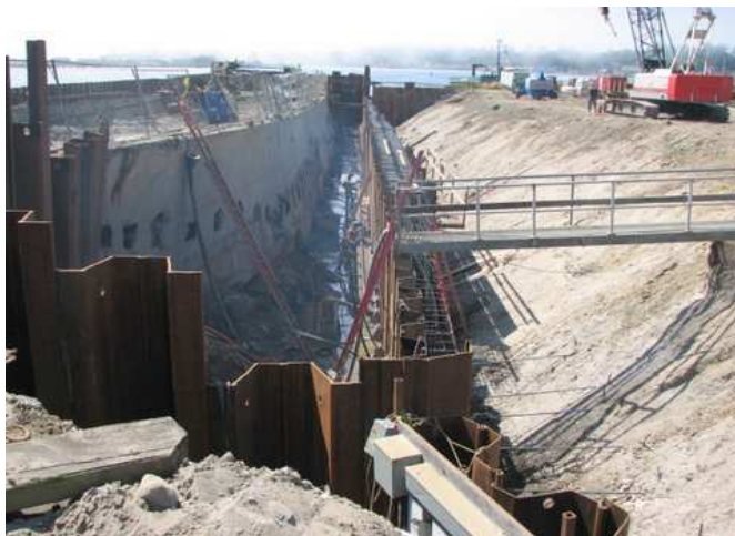
Permanent Bulkhead Retaining Wall at the SS Pasley
