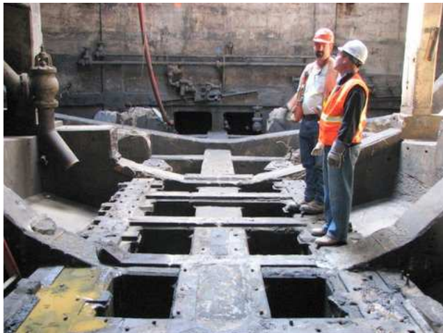
SS Hennebique Engine Room
