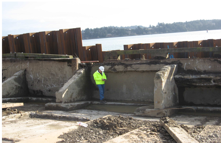
Working inside the containment cell around the Pasley
