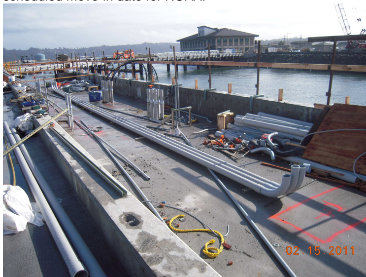
Work in progress on the NOAA pier
