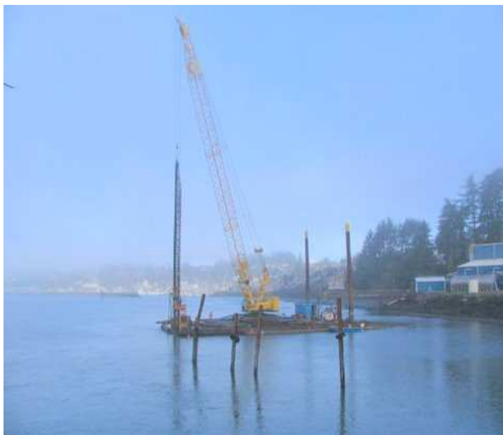
Pile driving at the Trident Meal Plant (Photo by Pete Dale)
