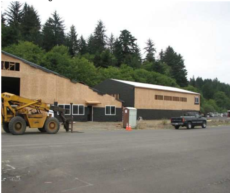
New Terminal Warehouse and Office Buildings
