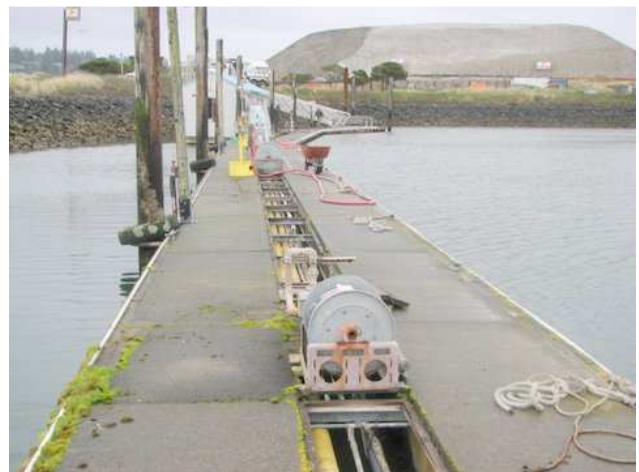
Fuel Dock work in progress
