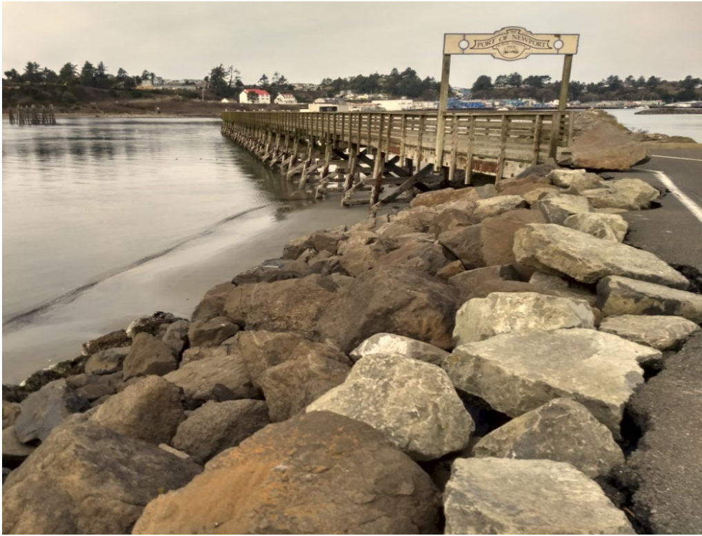
Photo 24 – Fishing Pier – Riprap
