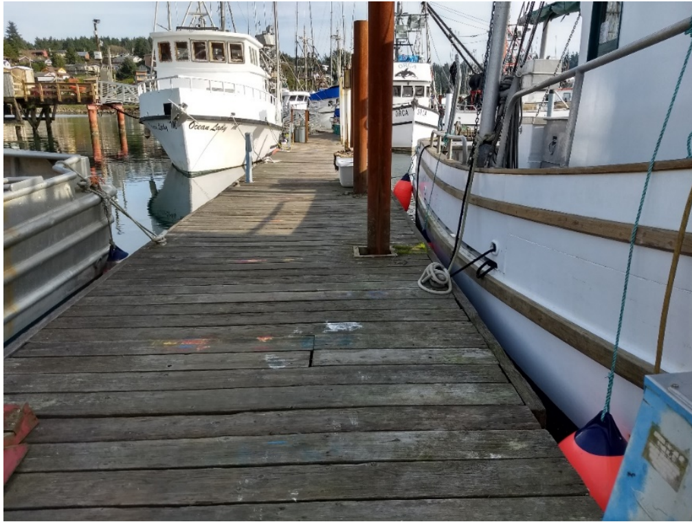
Photo 7 - Port Dock 5 - Wood Float
