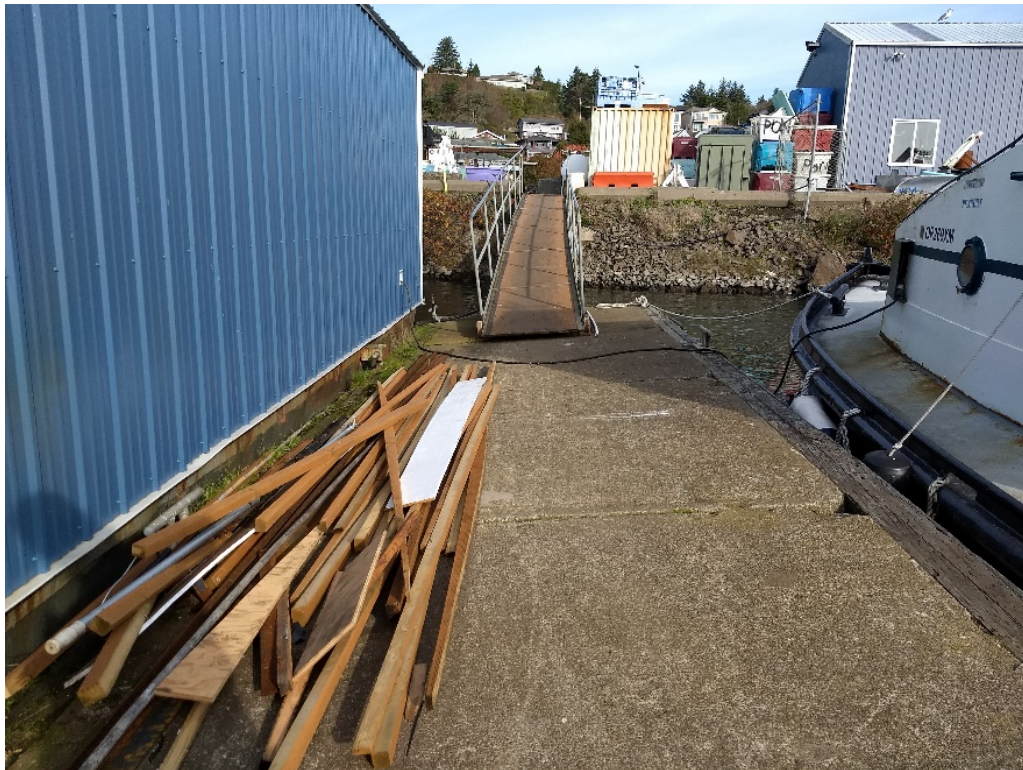
Photo 17 – Swede's Dock – Gangway and Concrete Float
